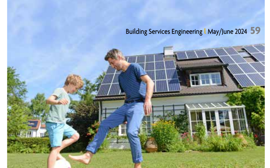
Rooftop solar installation is becoming increasingly prevalent.
