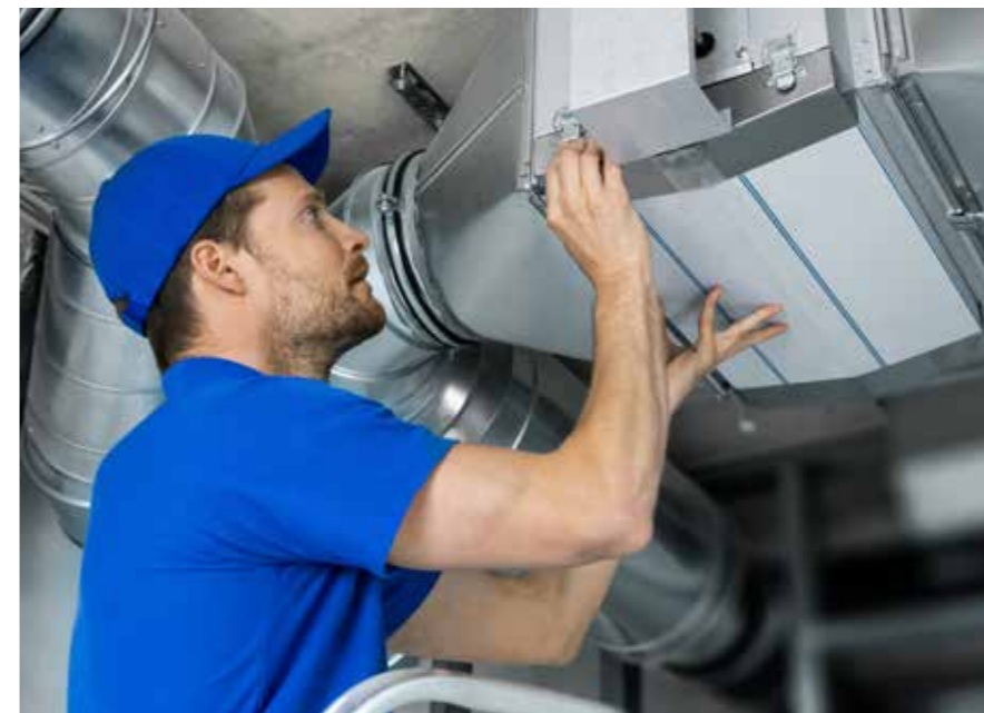
A ventilation system installation and repair service technician at work.
