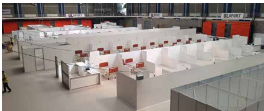
HTS were extensively involved in the planning, design and installation of services for the field hospital at the UL Arena in the University of Limerick.
